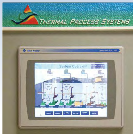
Control Panel — Delphos, OH An Integrated Control Package provides the flexibility to operate the processes by a simple touch on the screen.
