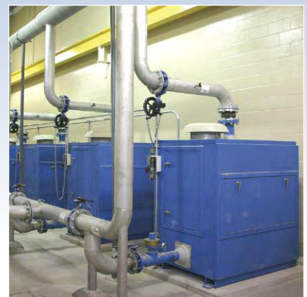
Positive Displacement Blowers — Delphos, OH Positive displacement blowers allow for the flexibility of varying the liquid depth in the reactors as well as air flow delivery.
