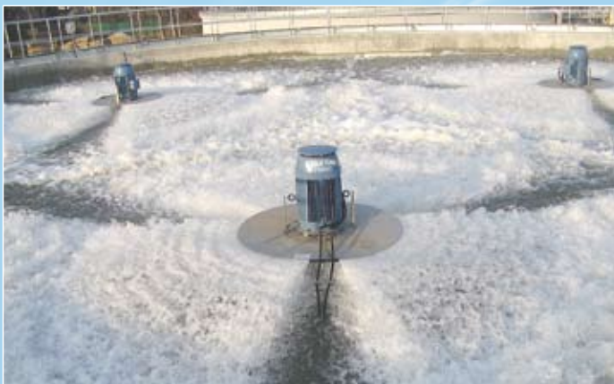
Spray and heat deflector
