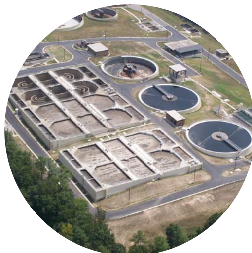
12.0 MGD BIO-DENIPHO with Secondary Anoxic Zones, North Cary WRF, Cary, NC
